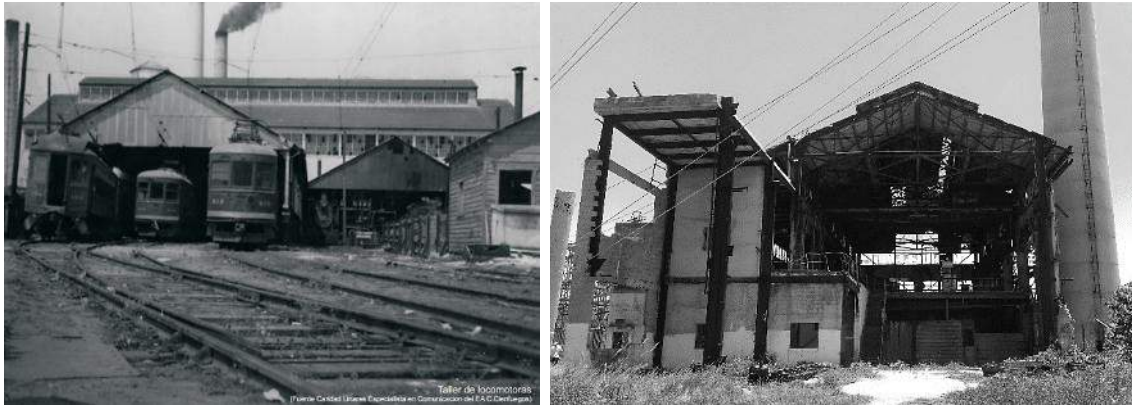
Figure 3.27 Railways workshop of Central Herhey.
