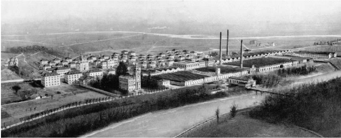
Figure 2.19 Crespi d'Adda and the surrounded landscape. It is possible to appreciate the hydroelectric and the channel
