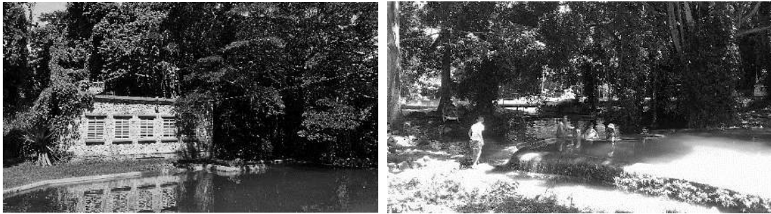
Figure 3.24 A small hydroelectric power station inside the natural park Hershey Gardens.
