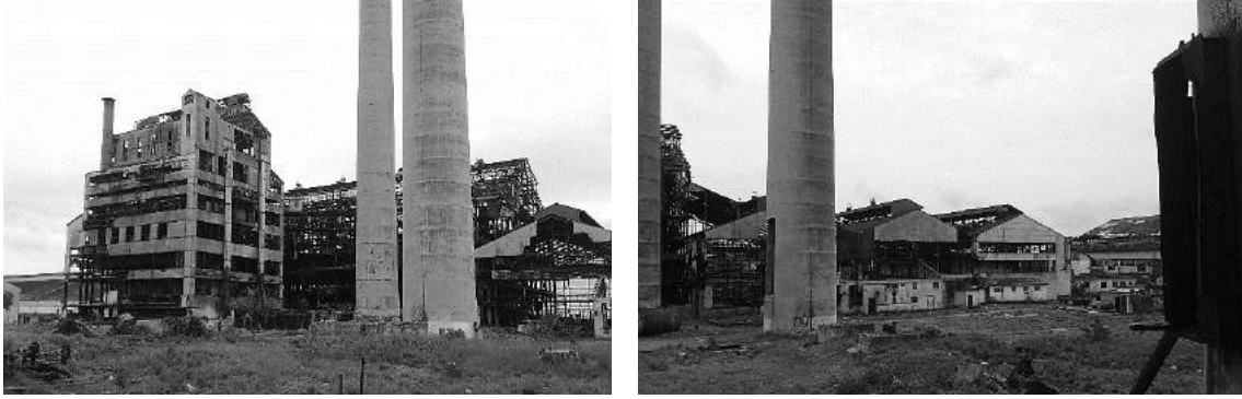
Figure 4.5 The coal house and the boilers house state before demolition.
