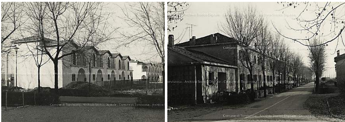
Figure 2.25 Image of the Colombaie houses in 1950
