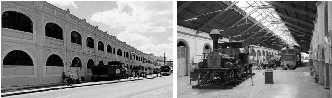
Figure 3.37 San Jose Warehouses in Habana Bay. In the exterior a recover old locomotive.
