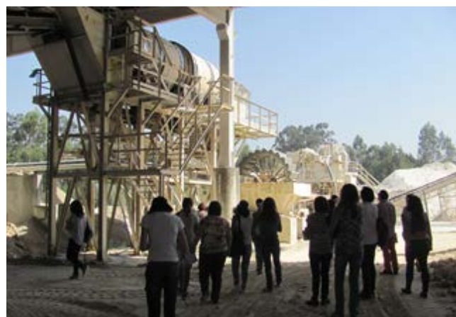
Figure 3. Kaolin treatment unit.
