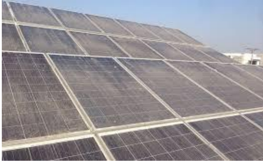
Figure 2.29 Dust on PV as time-independent obstacles.
