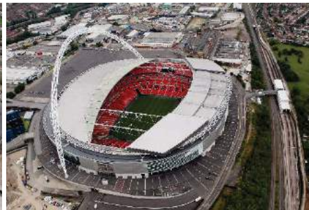
Figure 4. Wembley Stadium - Roof open
