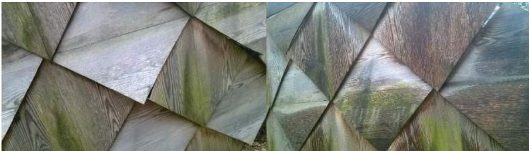
Figure 1. Ray 2 Responsive Wood Envelope Prototype a) in Semi-Dry April Weather When the Screen is Partly Open for Boundary Exchange between Exterior and Semi-Interior; b) After April Light Rain When the System is Closed, Not Allowing the Humid and Cold Air to Pass through the Boundary; both after Four Years of Being Exposed to Weather and Biotic Conditions. The prototype got inhabited by Blue Stein Fungi, Algae and Lichen. These, namely the algae, are regulating the moisture content of wood, thus co-causing its warping. Notice also the organisation of algae habitation caused by the material's fibre direction and position within the design that is affected by material performance and form. Thus it is organised through its moisture and the organism's abundance and distribution interaction (photos: Davidová 2017)
