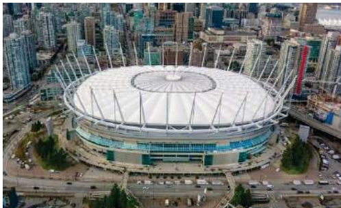
Figure 7. BC Place Stadium – roof closed
