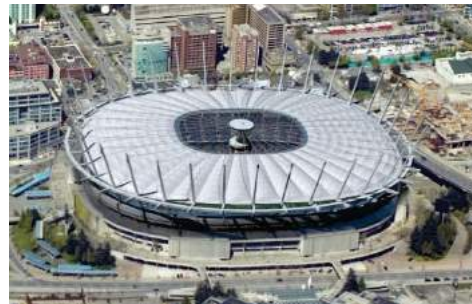
Figure 8. BC Place Stadium – roof open
