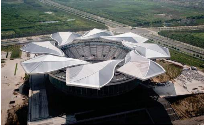
Figure 5. Qizhong Forest Sports City Arena - Roof open
