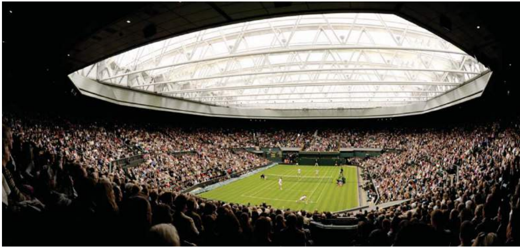
Figure 9. Wimbledon Centre Court – View from the inside, roof closed
