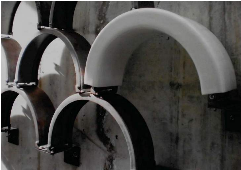
Figure 6. Lisbon Aquarium construction of the façade, Lisboa, Portugal. (Photodraphy by Campos Costa Architects).
