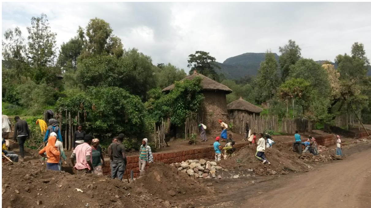
Fig. 3.3. Repaving the "Honey street"
