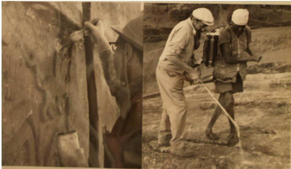
Fig.2.7. Angelini’s workers using chemical in the church of Medhane Alem
