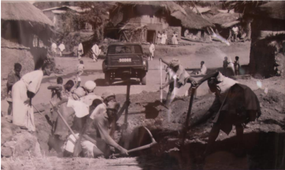
Fig.2.8. Angelini's workers digging the trenches
