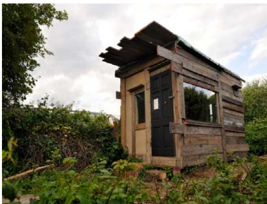
i57. Grow Heathrow. Oliver Lowrie, Rocket House . 24 parafusos de metal 400 parafusos de madeira 2 rolos de lã de rocha 100 £
