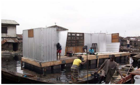
i74. Architecture for Humanity. Makoko Amphibious Clinic , Lagos, Nigeria (2009).
