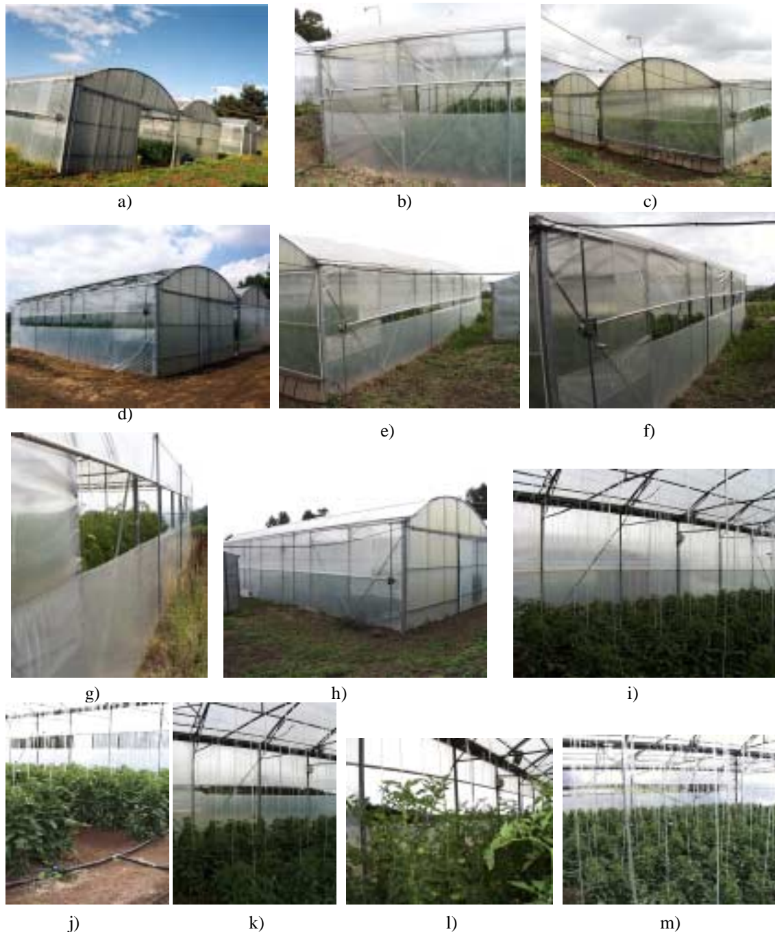
Figure 2.7 – Different views of the ventilation apertures of permanent and classical ventilated greenhouses: a) general view of the greenhouses, b) side opening 54 cm, c) cables connecting inside sensors and data loggers, d) side and roof openings, e) side opening 22 cm, f) detail of the rolling system, g) side opening 75 cm, h) external view of the night closed greenhouse, i) internal view of the night close greenhouse, j) internal view with side opening 54 cm, k) internal view with side opening 22 cm, l) internal view with side opening 75 cm, m) internal view with plant tutors
