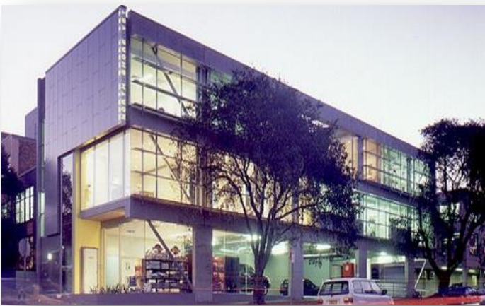
Fig.1 - North Shore Veterinary Hospital building
