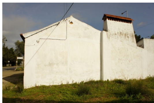
Fig.4. Monitored facade (West facade).
