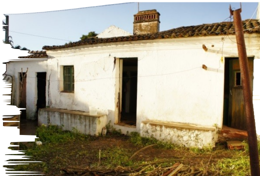
Fig.1. Monitored facade (South facade). probes' location.
