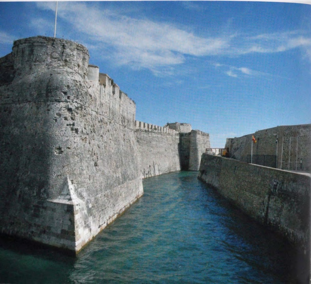
Fig 1. Fortress of Ceuta. Bastioned front land, built in the 1540's. Photograph from the author.
